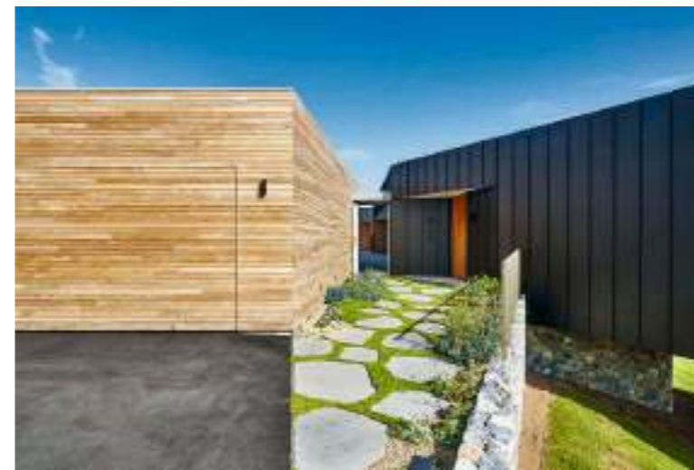
Below: The wood from local eucalyptus trees contrasts beautifully with the black aluminium façades.
